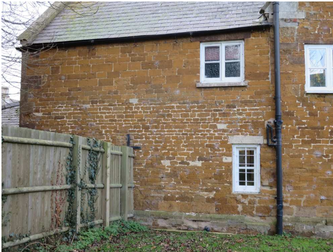
The rear east wing, with added first floor – note straight joint beside downpipe
