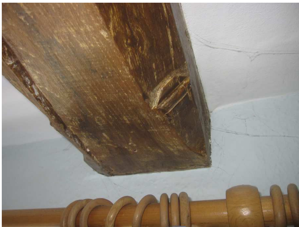
Chamfer stop to ceiling beam
